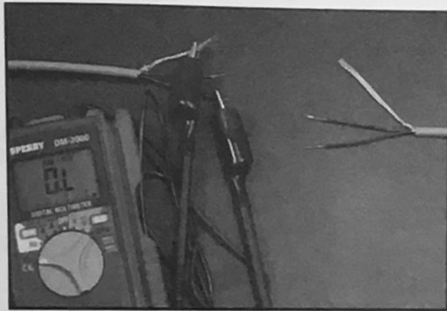
Step 2.8. Use a digital multimeter and a TDR to test from this location. Check for any additional cable damage by "looking" down the cable in both directions. For assistance in using these test instruments, consult the instructions that came with them or contact Watts Radiant.
